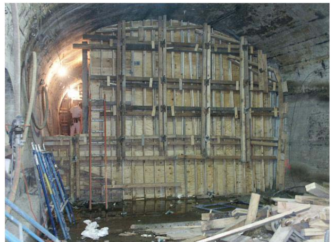
Fig.10 Formwork for Tunnel Backfilling
