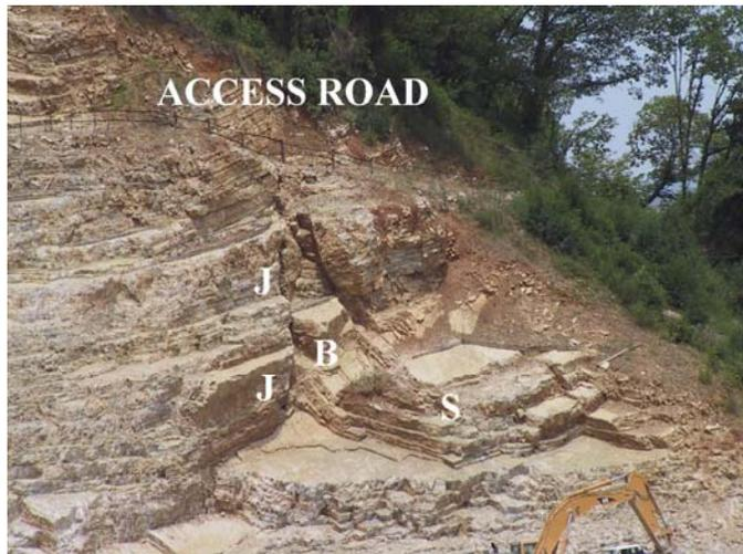
Fig. 2 Picture taken on 25<sup>th</sup> June 2003 of the collapsed rock mass before the failure: JJ sub-vertical joint, B Block, S 20° dipping stratification)
