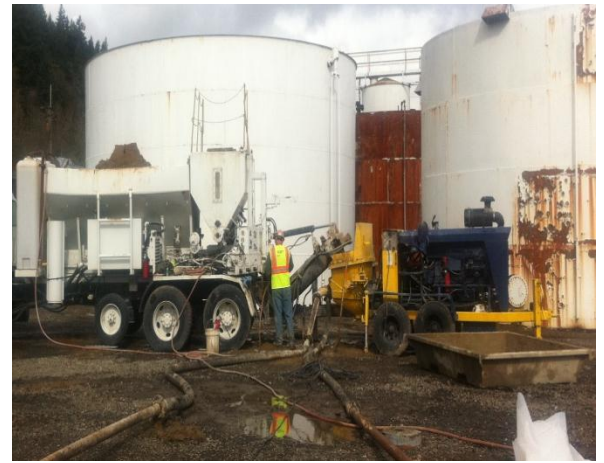
Fig. 14. Mixing grout using a continuous mixer
