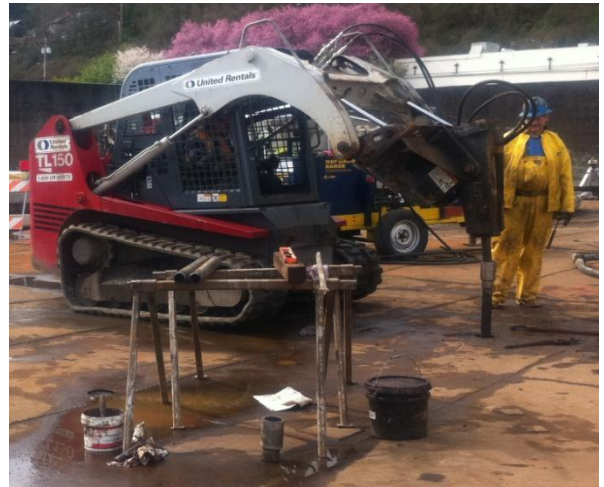
Fig. 13. Installing casings by driving using a limited access rubber track rig
