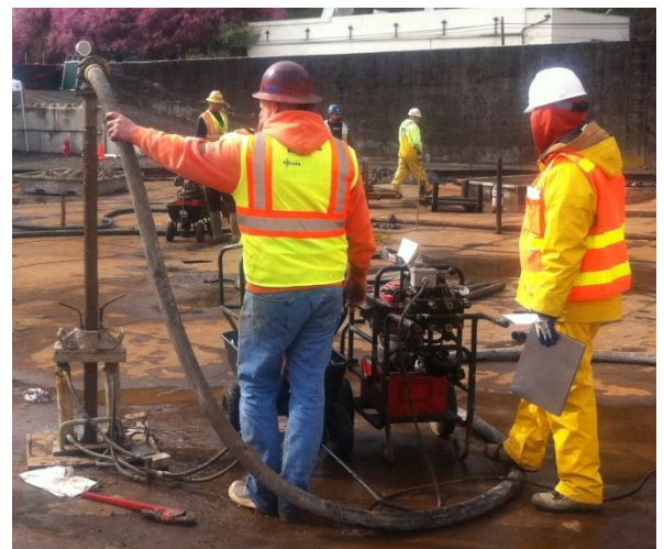
Fig. 15. Compaction grout header and the duplex jacks for casing extraction
