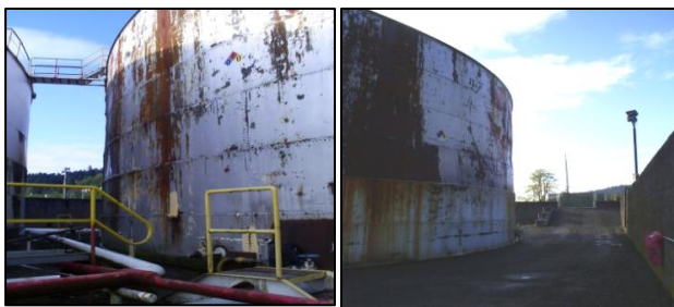
Fig. 3. Surface Conditions (looking west and southeast)
