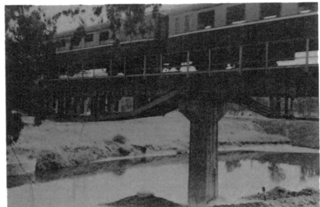
Fig. 2 - Eastward view of pier 2.
