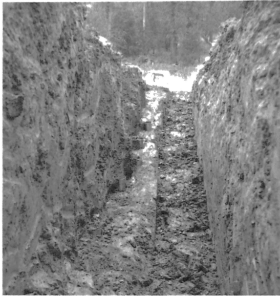
Fig. 5. Downslope View of Trenched Slide Showing Exposed Slide Plane.
