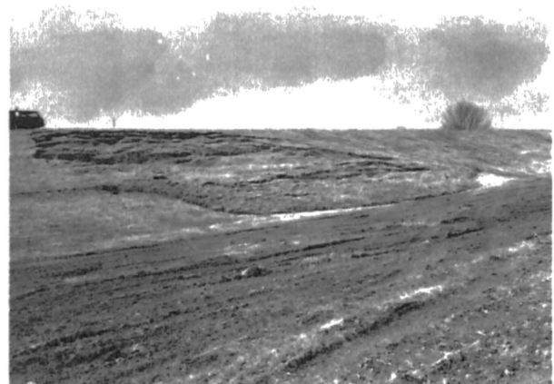
Fig. 1. Typical Levee Slough Slide.
