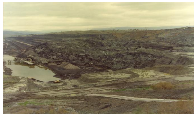
Fig.6: General view of the slope failure.
