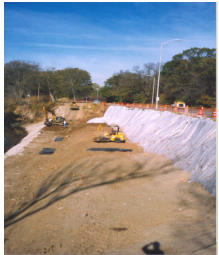
Fig. 7. Blue River construction aspects
