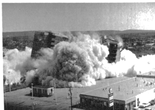
Fig. 9. Building Just After Demolition
