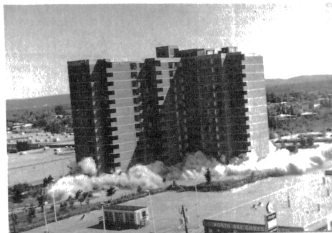
Fig. 8. Building Just Prior to Demolition
