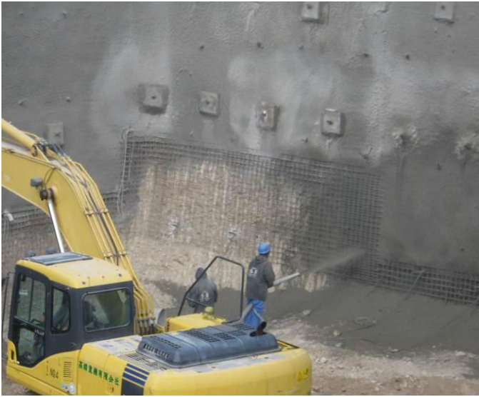
Fig. 12. Construction sequence: Temporary facing using steel mesh and shotcrete
