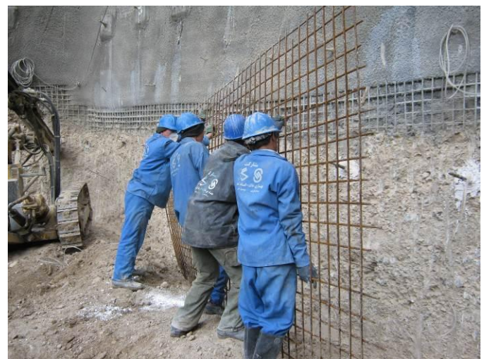
Fig. 11. Construction sequence: Temporary facing using steel mesh and shotcrete
