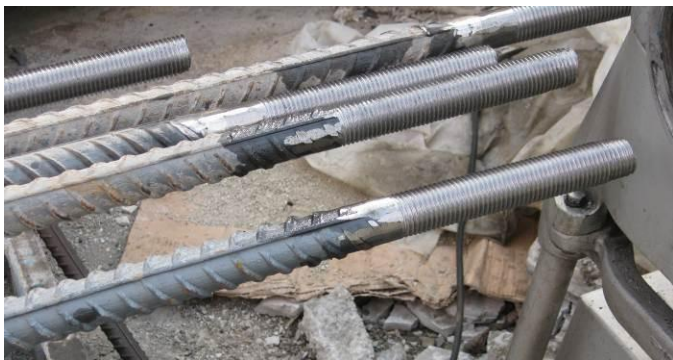
Fig. 9. Steel bars are threaded so that a heavy duty nut can be fitted to the nail head
