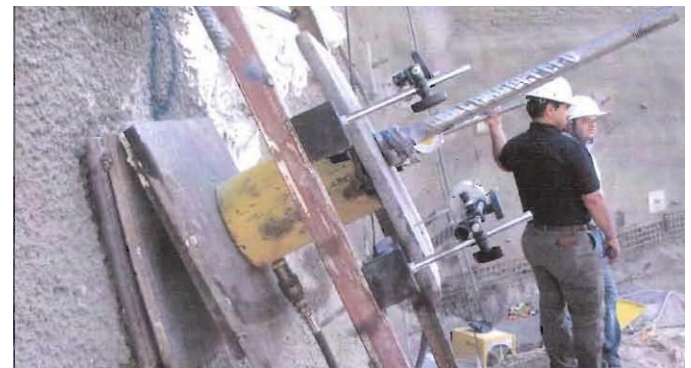
Fig. 21. Pull out test apparatus at the site
