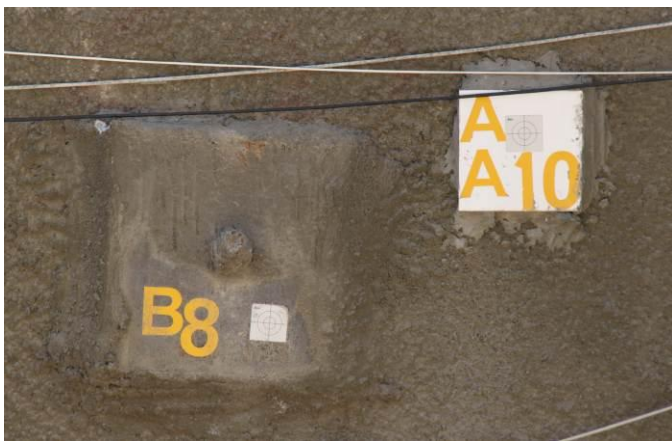
Fig. 23. Targets installed on the shotcrete facing and nail heads
