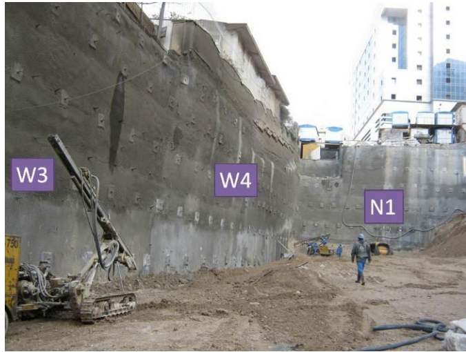
Fig. 16. W3, W4 and N1 soil nail walls during the excavation process
