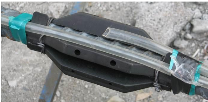
Fig. 8. The centralizer and the injection pipe attached to the nail
