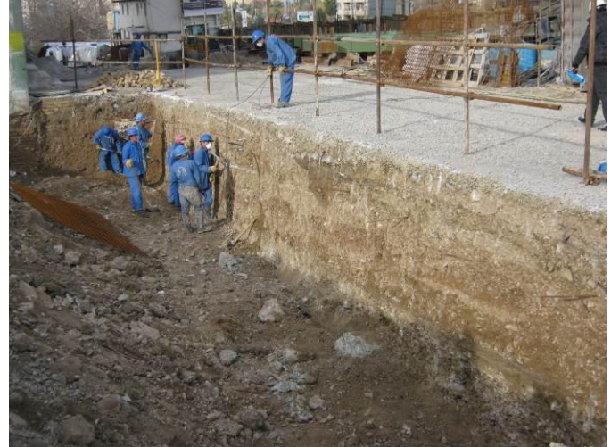
Fig. 6. Construction sequence: Excavation to a stable depth
