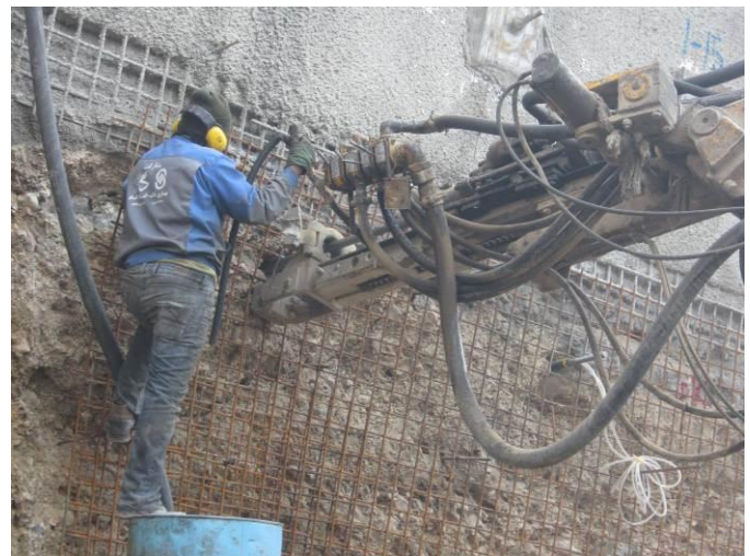
Fig. 7. Construction sequence: Installation of soil nails - Drilling
