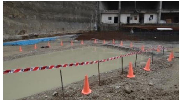
Fig. 25. Accumulation of precipitation water in an excavated pond
