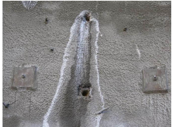
Fig. 28. Finished surface after installing the drains
