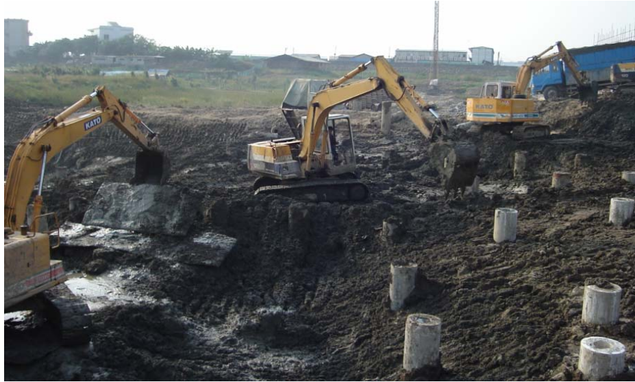
Fig. 5 Photo of construction activities following the recommendations
