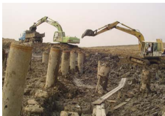
Fig. 2 Severe inclination observed during excavation a) photo during construction; b) illustration of pipe pile inclination
