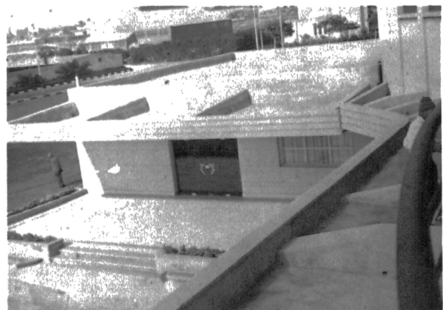
Fig. 1. A Front Elevation Photograph showing The Annexe and its Connection with the existing Main Building.
