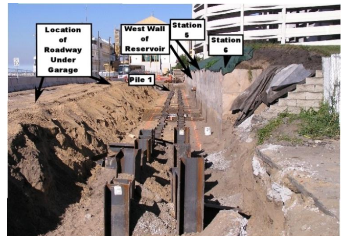
Fig. 7: Driven piles and West wall of Water Reservoir.
