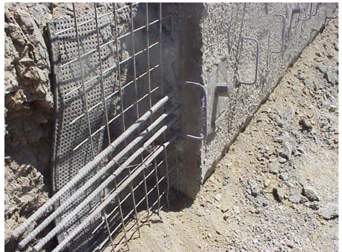
Photo 5. Primary Wall Section
