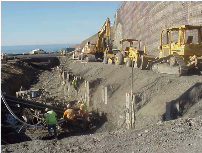
Photo 10. Installing a Sheathed Tieback Anchor in a Drilled Hole
