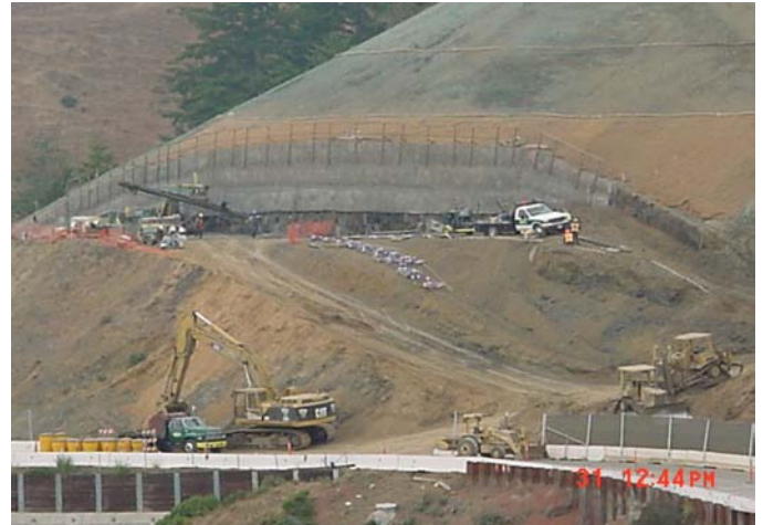
Photo 4. Soil nailed Wall Construction at 4 th Lift
