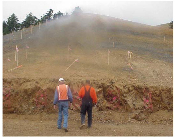
Photo 3. Graded Slope above Soil Nail wall and 1 st Exc. Lift
