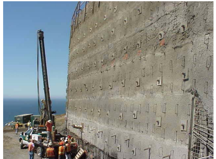
Photo 6. Setting up a Soil nail Test
