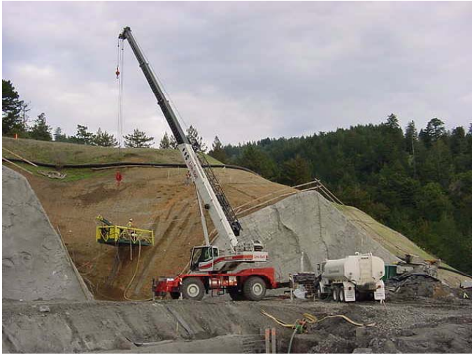
Photo 11. Drilling for Return Walls on Side Slopes
