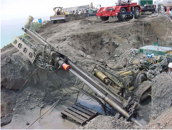
Photo 9. Drilling between double beams for tieback Wall
