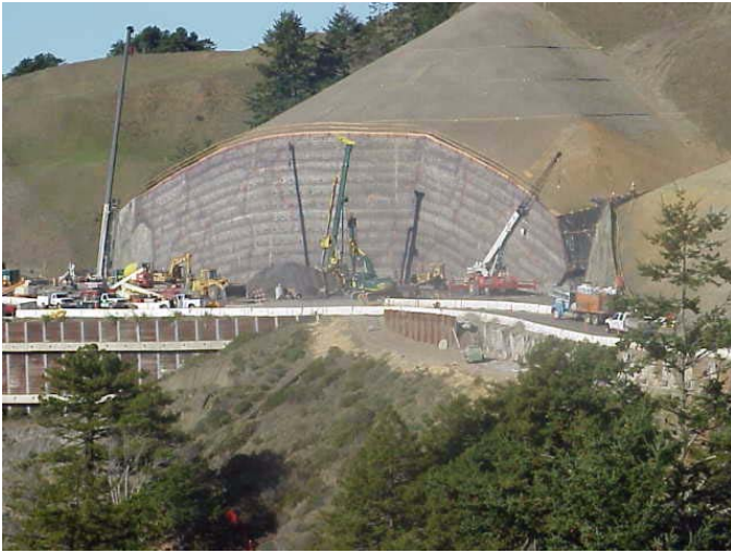
Photo 8. Completed Soil Nailed Wall with Primary Facing
