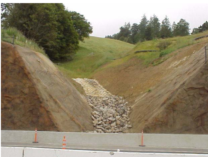
Photo 12. Creek Return Walls and Rip Raps Slope Protection
