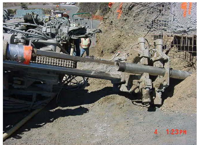
Photo 7. Drilling on north side of Soil Nailed Wall Using Casing
