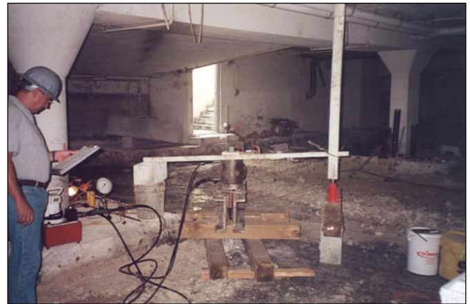
Photograph J – Anchor load test set-up
