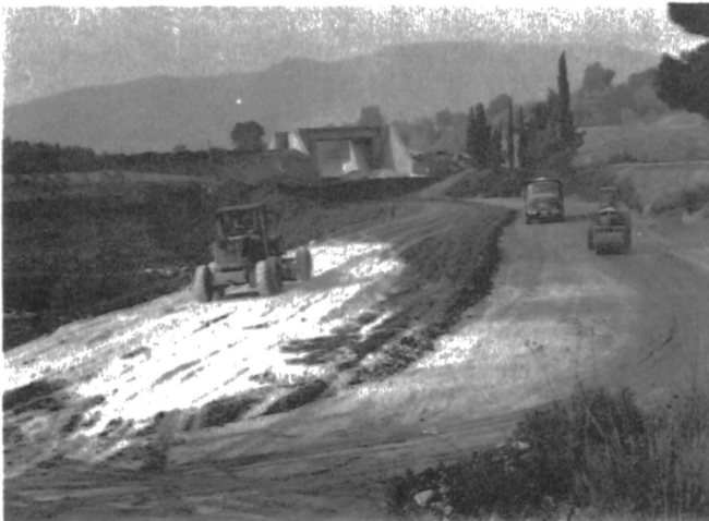
Fig. 4. Soil-Lime Mixing by Grader
