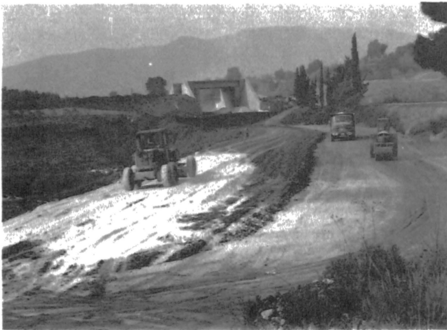
Fig. 4. Soil-Lime Mixing by Grader
