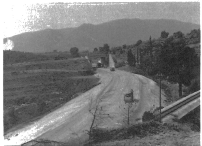
Fig. 5. Final Leveling of Embankment with Selected Crushed Material
