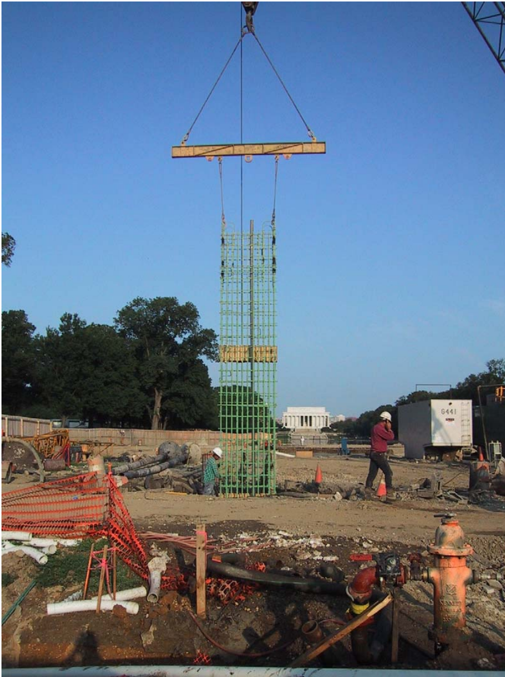
Fig. 10. Reinforcing cage being placed for WWII Memorial Slurry Wall (2002)
