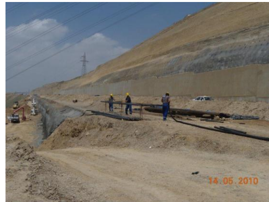
Fig. 6a. Cut Slopes-Drainage and nailing
