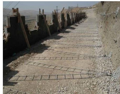
Fig. 9. Construction Phases – Galvanised Steel Ladders
