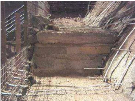
Fig. 5. Friction Connection with Galvanized Steel Ladder Strips
