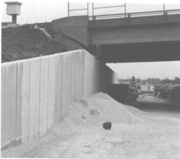
Fig. 4 Completion of Wall A5316 at Lindbergh Boulevard
