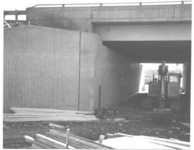
Fig. 7 Completed Retaining Wall at Truman Drive
