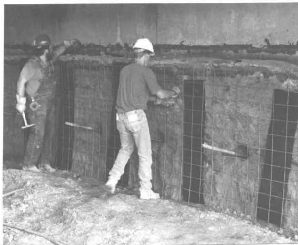
Fig. 3 Construction of Temporary Wall at Lindbergh Boulevard
