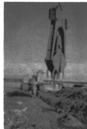
Figure 3. Installation of slurry trench and sheet-piles.
