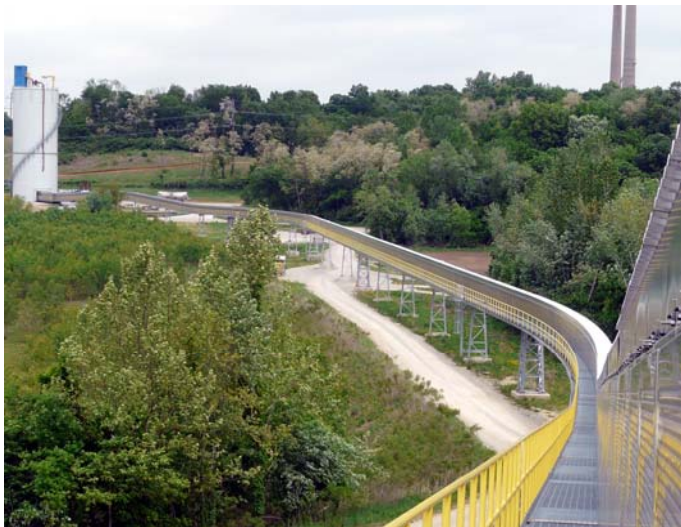
Fig. 3. Storage Silo and Tubular Conveyor.
