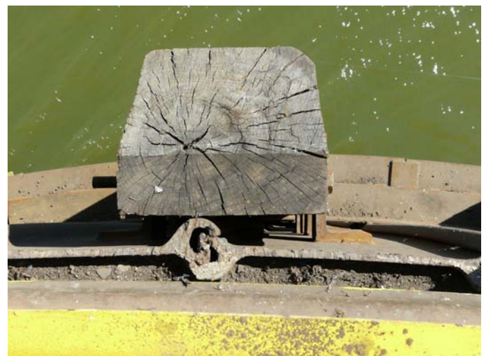
Fig. 12. Installed timber fender.
