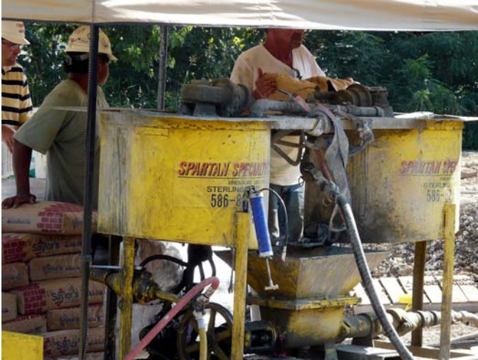
Fig. 19. Site mixed grout plant.
