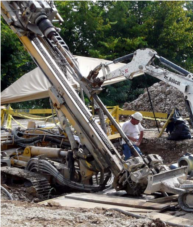
Fig. 17. Klemm duplex drilling system rock anchor drill.
