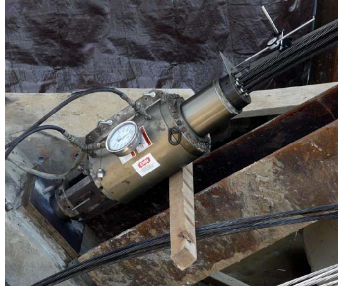
Fig. 20. Anchor stressing jack cylinder.
