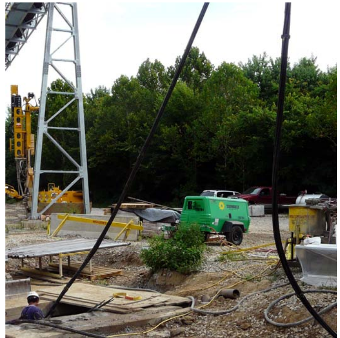
Fig. 18. Anchor tendon installation.
