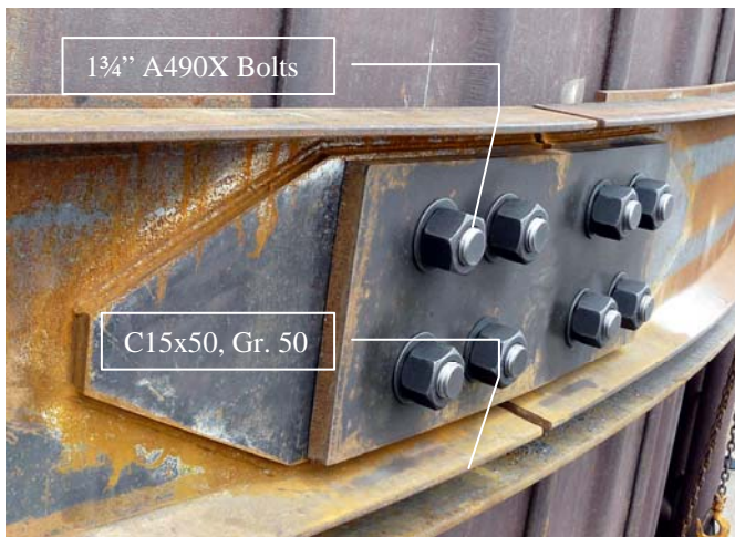
Fig. 7. Tension Belt Channel Splice.
