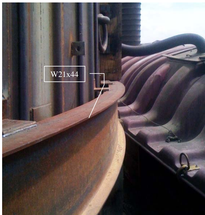
Fig. 10. Protective W21x44 section.
