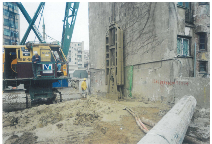
Photo 6. The slurry wall execution - front image
