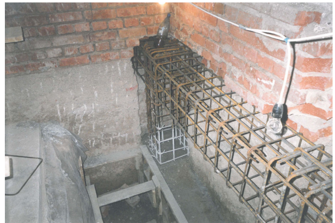
Photo 10 New foundation reinforcement inside the church
