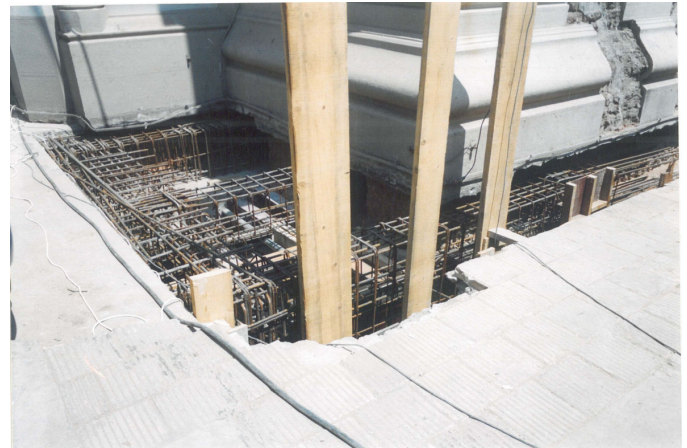
Photo 9 Supplementary foundations area near the church entrance
