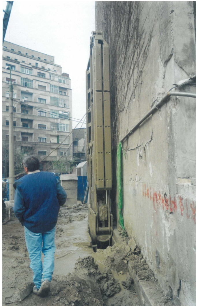
Photo 5. The slurry wall execution - lateral image
