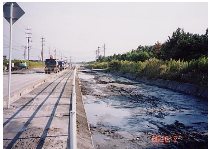
Photo 5. Liquefaction-induced flow toward a small river
