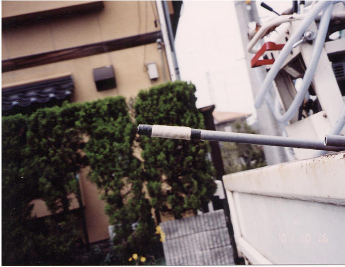
Photo 6. Vinyl tube with strainer to measure depth of groundwater level
