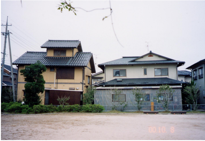
Photo 1. Settled and tilted houses due to liquefaction in Abehikona development
