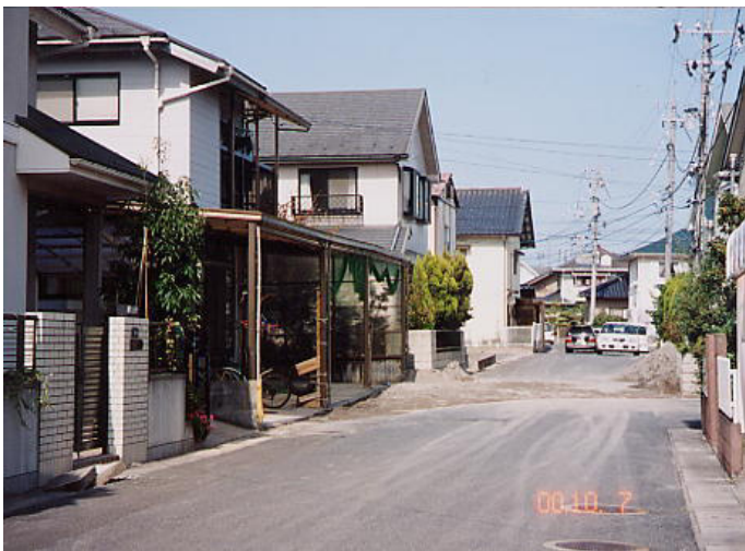
Photo 2. Boiled sands in Abehikona development
