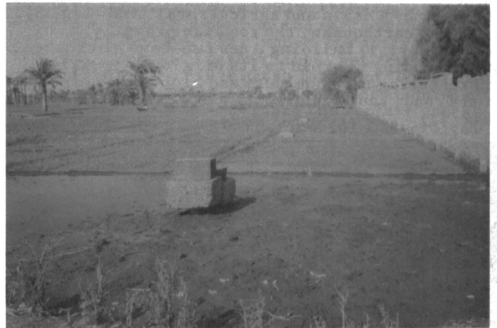
Fig. 10a. An abandoned steel pipe covered with a concrete block moved upwards relative to the surrounding soil.
