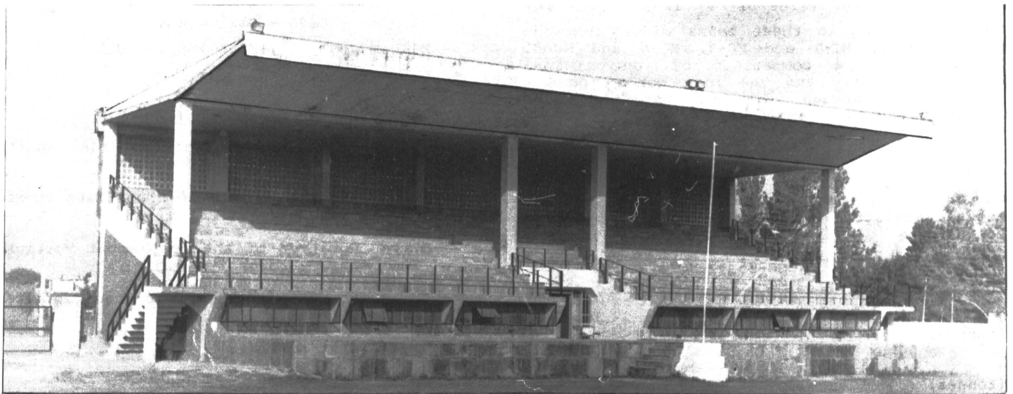
Figure 6 - A View of Finally Constructed Stadium Building.
