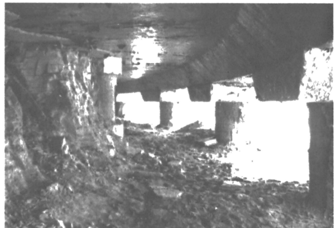
Fig.17. Creation of void under cooling tower ponds by undermining.
