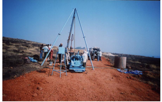
Fig.1. Geotechnical Investigation at Site
