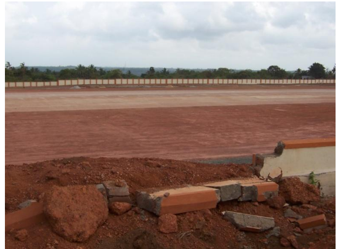
Fig.16. Proper compaction at site is very important for highway and airport runway pavements
