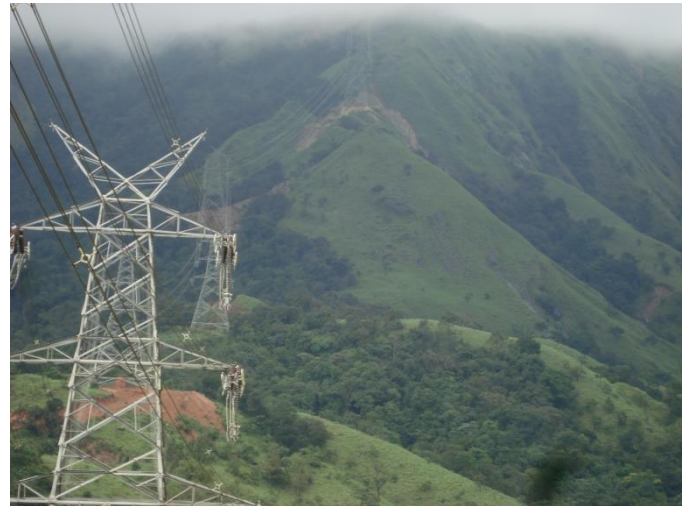
Fig.3. Example of extremely difficult and remote places for geotechnical engineers to work. Land slide in a distant hill slope can be seen which also houses a transmission tower
