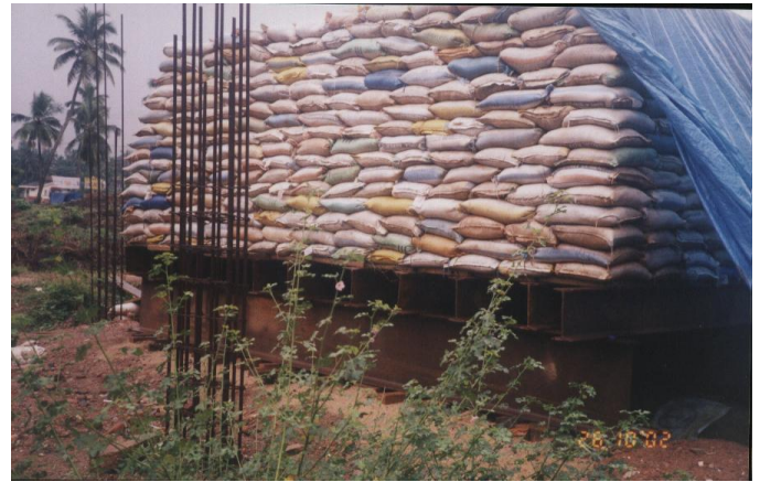
Fig.2. Field Load Testing using kentledge loading
