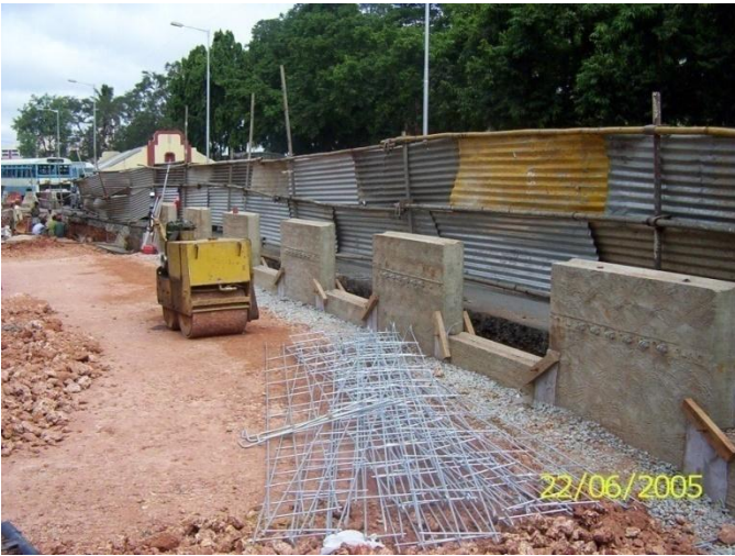
Fig.15. Compaction for an approach embankment to a flyover
