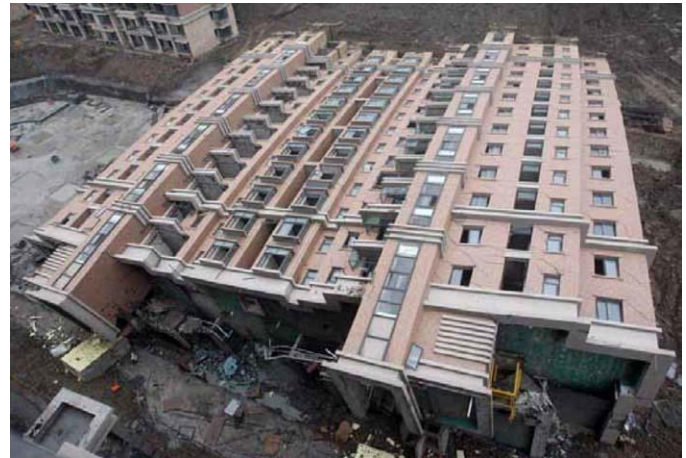
Fig.6. View of building after failure (Subramanian, 2009)
