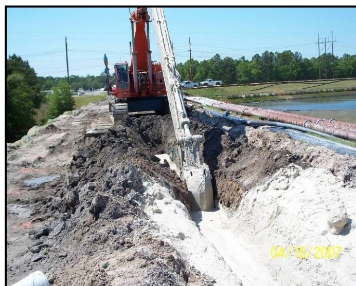
Fig. 5 Construction of the CB slurry trench.
