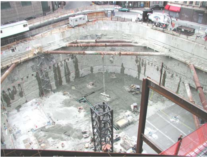
Fig. 9. The Arched Slurry Wall
