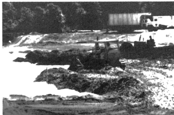
FIGURE 7 - CONSTRUCTION OF WORKING PLATFORM WITH WOOD CHIPS
