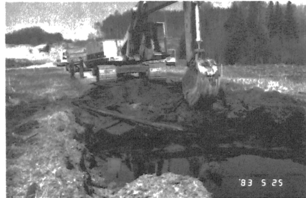
FIGURE 11 - EXCAVATION OF EXISTING ROAD FILL
