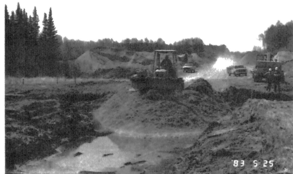
FIGURE 12 - REPLACEMENT WITH WOOD CHIPS
