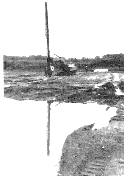
FIGURE 3 - INSTALLATION OF ALIDRAINS AT EDEN PRAIRIE PROJECT
