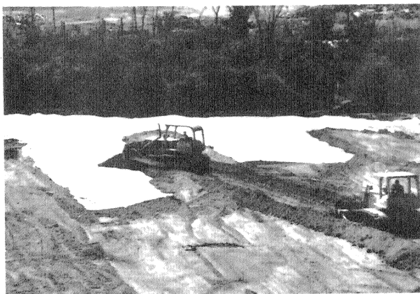
(b) PLACEMENT OF SECOND SYSTEM STRIP EMBANKMENTS
