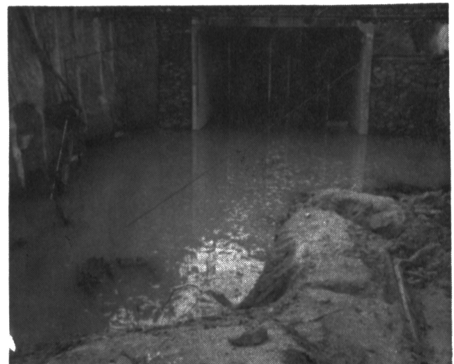
Fig. 2 Water Inflow during Constructive Process
