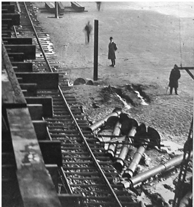
Fig.8. Work in progress at Weston Pier.
