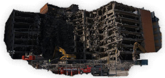
Fig. 2. Demolition of 7 to 9-story Parking Garage
