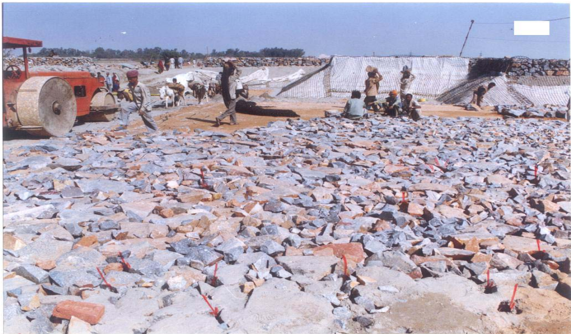
Fig.6(b). Photo plate showing the geo fabric, overlaying rope mattress and stone
