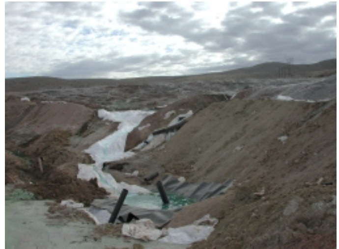
Fig. 5. Liquefaction-related damage at the Locumba bridge site.
