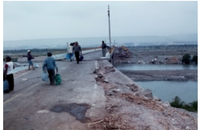
Fig. 11. El Fraile Bridge, damaged by liquefaction, was closed to vehicular traffic. A collapsed structure is faintly visible across the river to the right of the bridge.
