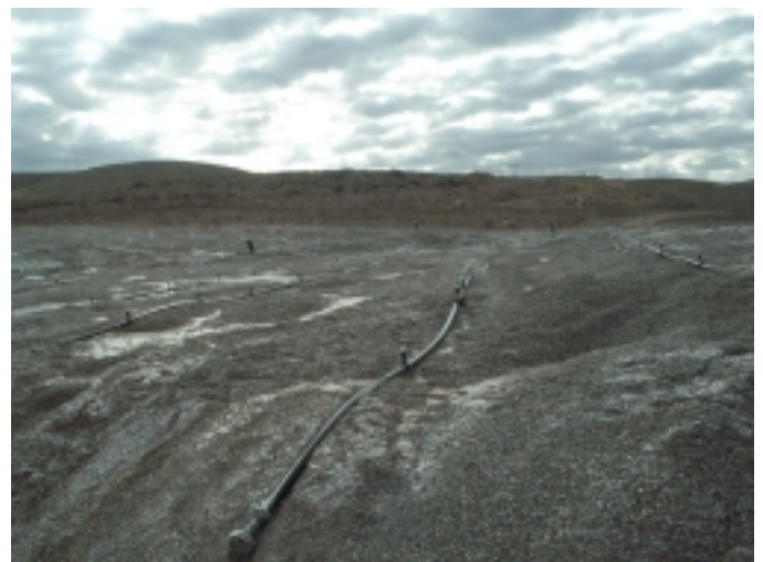
Fig. 7. Failed heap leach pad at Cajone mine.
