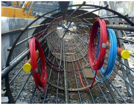
Fig. 16. Reinforcement cage with attached tubes and measuring equipment
