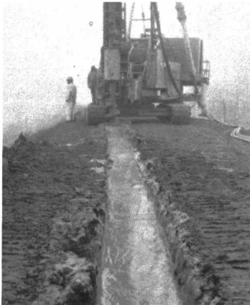
Fig. 13 View of SMW Work on Levee
