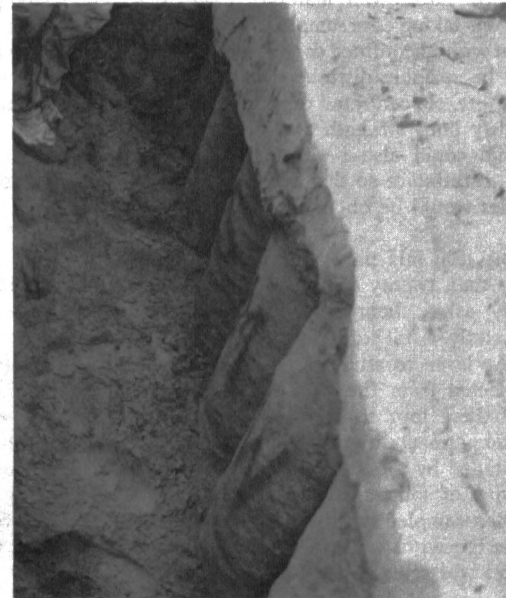
Fig. 14 Exposed SMW Columns
