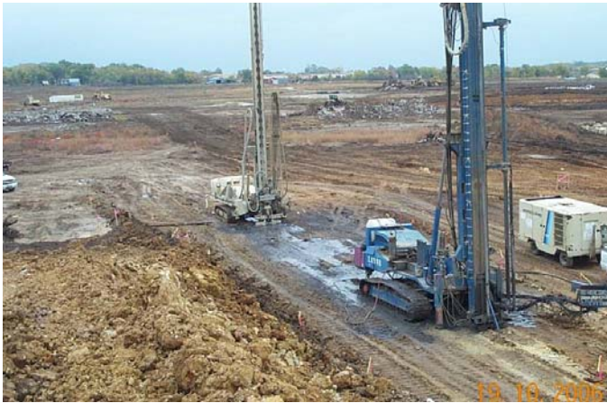
Fig. 3. Typical Ground Treatment Process – One rig drilling, one grouting
