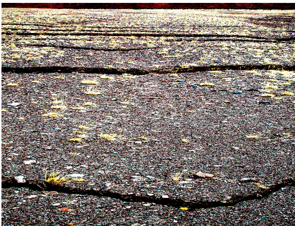
Fig. 9. Seismic subsidence caused ladderlike stripes in the North of the Kusai Lake
