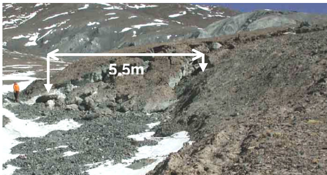
Fig.6. Horizontal displacement caused by the 8.1 great earthquake
