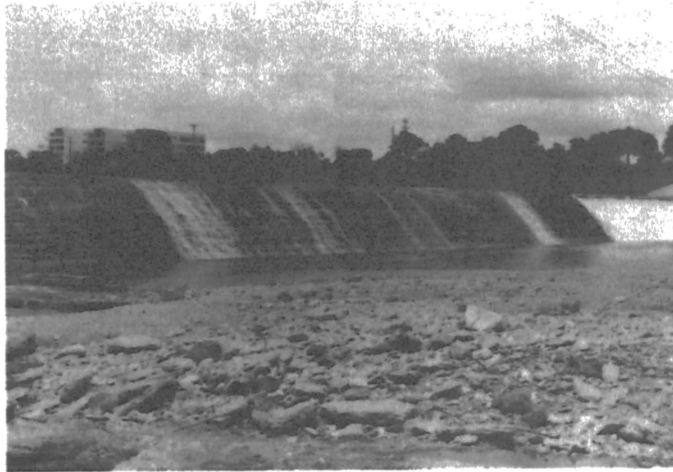
Fig. 9 Completed Dam, July 1987
