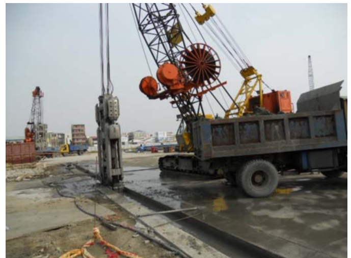
Fig. 15. Installation of Slurry Wall - Tainan
