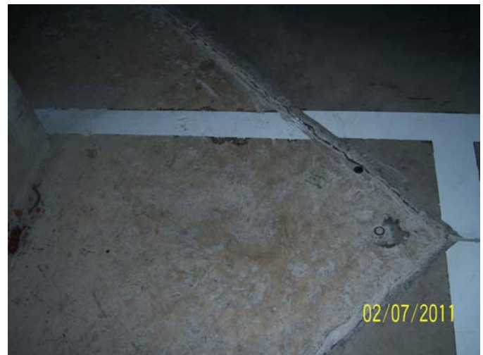
Fig. 9. Repaired Joint - Taichung
