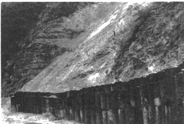
FIG. 6 DRUM DIAPHRAGM RETAINING WALL ON KALIASAUR LANDSLIDE
