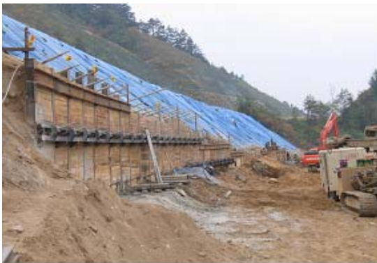
Pic.5 Temporary retaining wall
