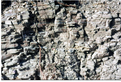
Fig. 4. Photo showing desiccated Clay Profile.
