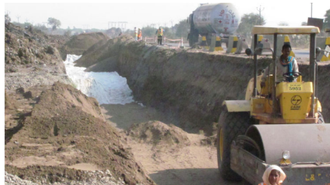
(b) Laying of geotextile
