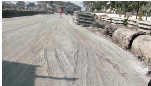
(a) Flyash mixing for soil stabilisation
