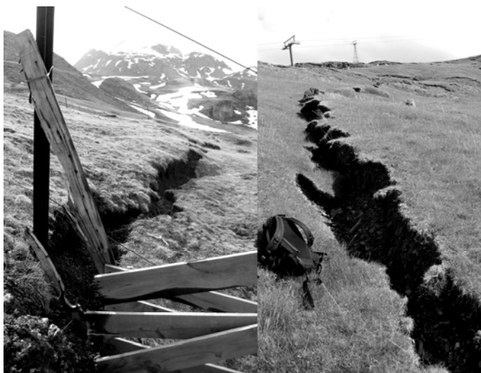
Figure 2. Cracks at the crest of the slide.
