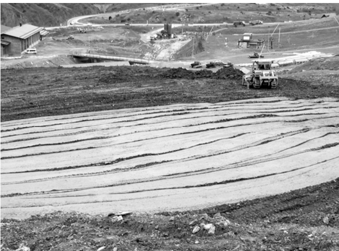
Figure 11. Placement and compaction of fill material
