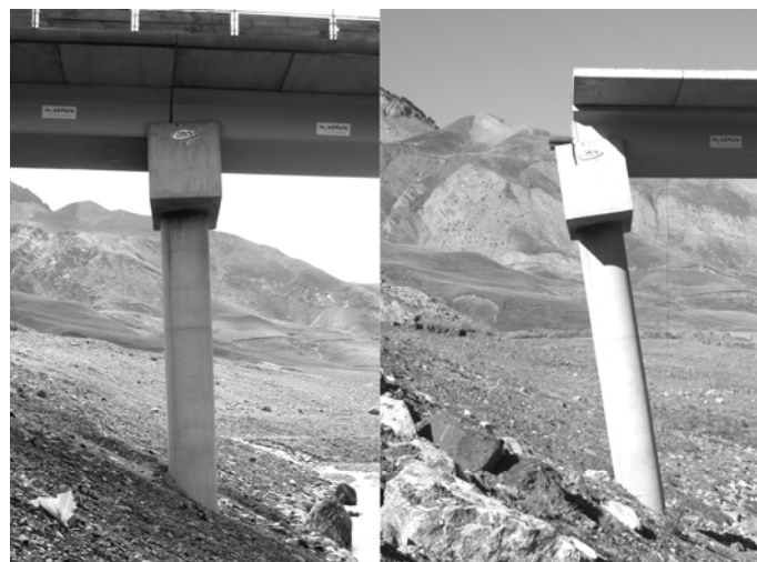
Figure 3. Evolution of the movement of a pillar located close to the toe of the slide
