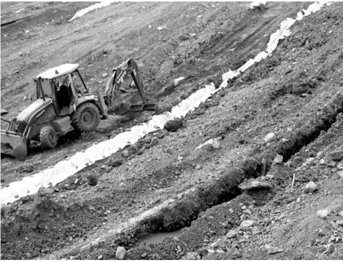
Figure 10. Construction of the drainage trenches
