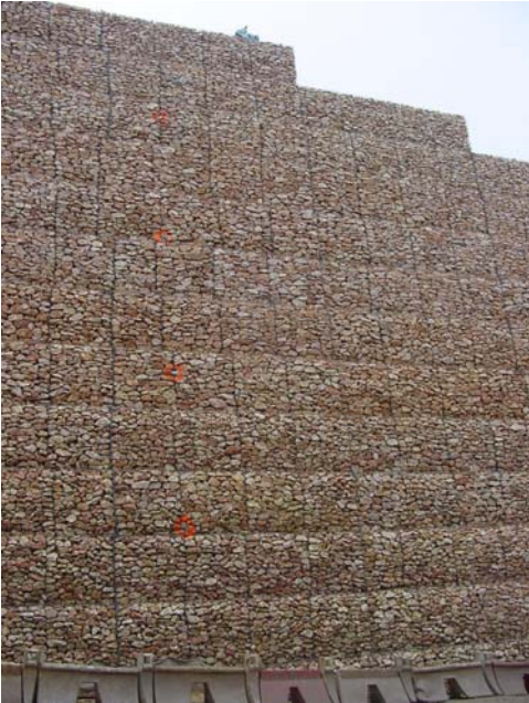
Photo 1. General view with backfill
