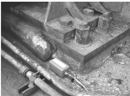
Figure 3. A sensor installed at the driving end of Fan 1-B
