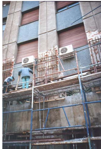
Fig. 9 Photo during the execution (axis “1”)
