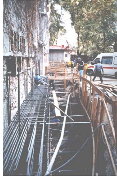
Fig.8 Photo during the execution of the foundation beam (axis “A”)
