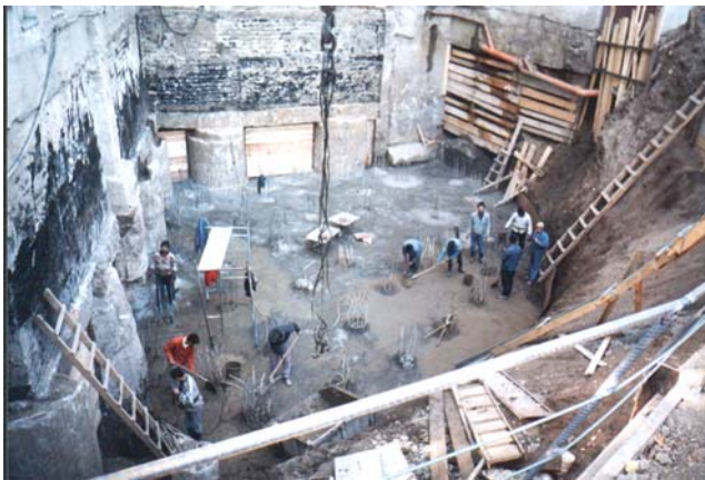
Fig. 7 Photo after the execution of the piles
