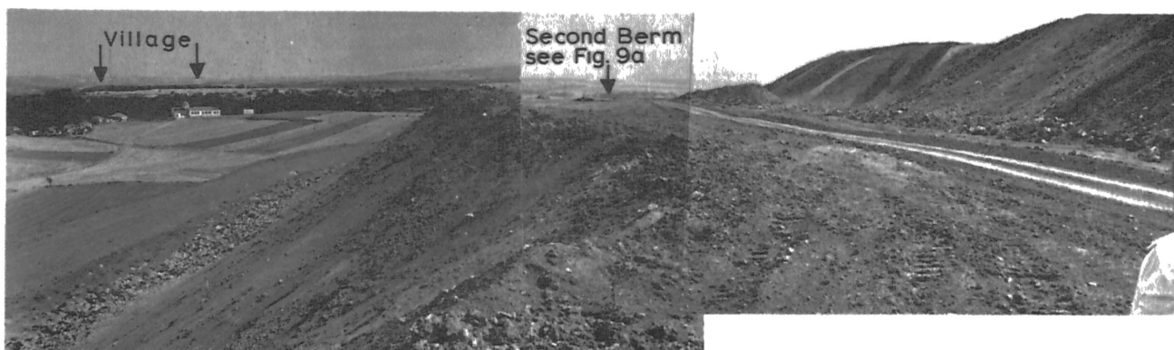
Fig. 1. View of Fill at the Time of Investigations
