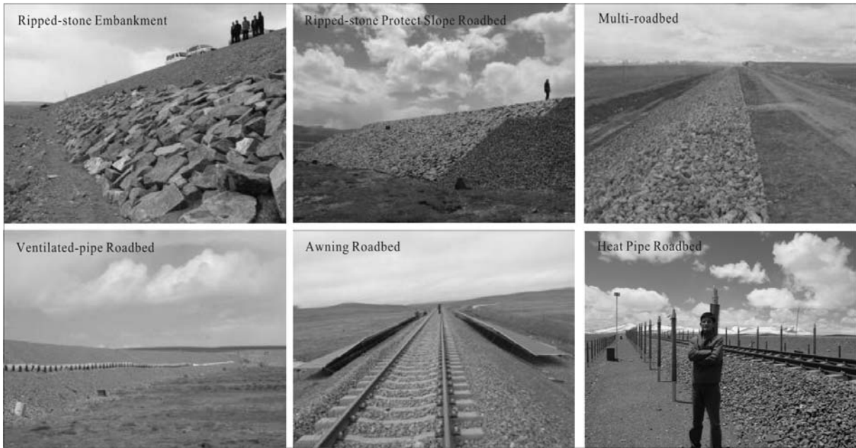
Fig. 6. Examples of Engineering Measures Applied in QTR.
