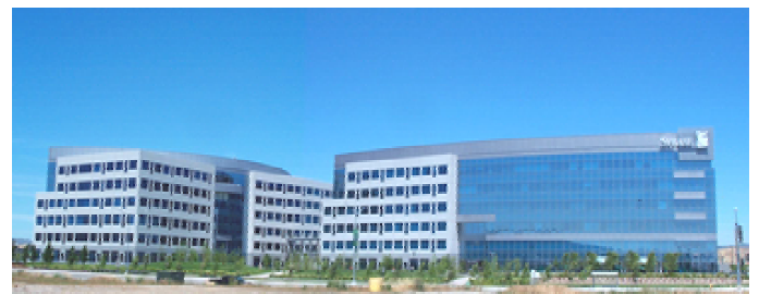
Fig.3. 6-Story Class A Offices in Dublin, CA
